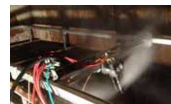
CONDENSER TUBE CLEANING
